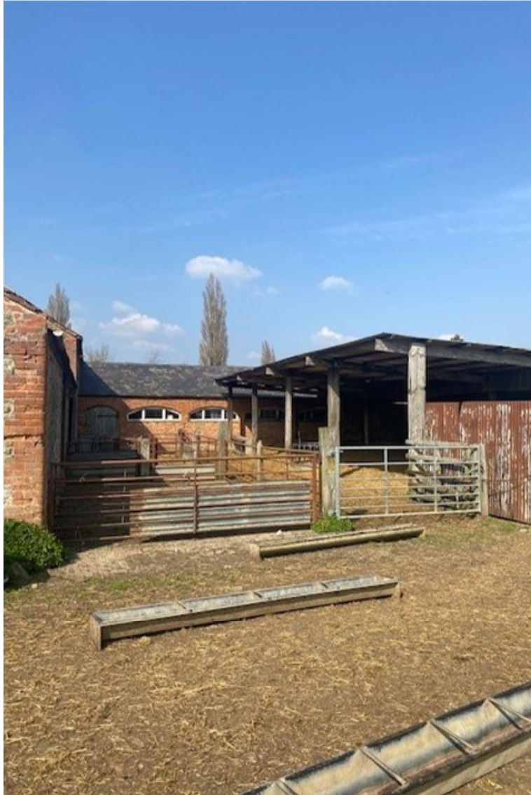
P3. Looking north east
