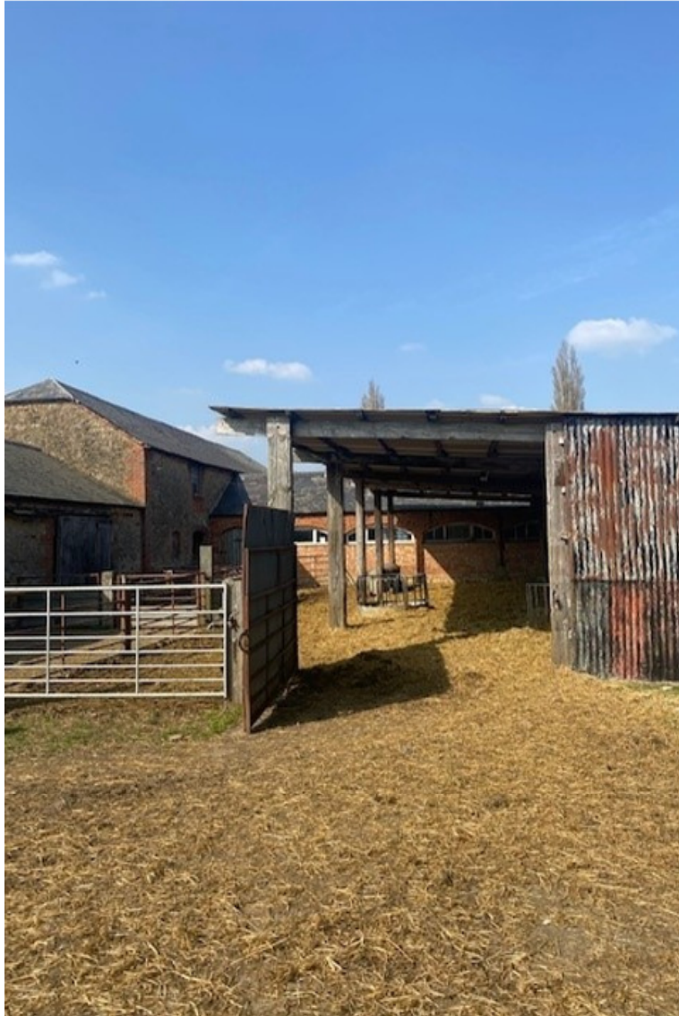
P1 - Looking north
