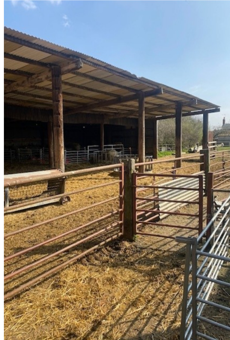
P2 - Looking south
